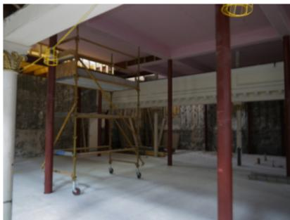
support the upper floor; the steelworks were erected; the ground and upper flooring was laid; the whole area underneath the upper floor was covered with a double layer of fireboard which also encases the steel beams; the baptistry was formed; and on the ground floor the foundations for the lift shaft and the fire escape are built and initial plumbing works completed.
